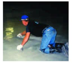
After Coca-Cola's old epoxy mortar floor system was removed with jack hammers, the exposed concrete substrate was mechanically prepared. After prepara tion, Stonhard's specially trained installation team screed applied a four-component urethane mortar with quartz aggregate broadcast for texture. This was followed with a high performance urethane seal er for an extra measure of chemical and abrasion resistance.
